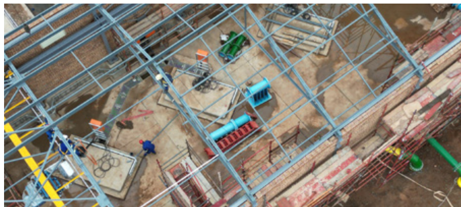
📷 Construction in progress at Spitskop Pump Station 2.
