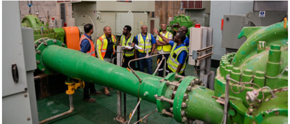
Team members inspecting Havercroft Pump Station.
