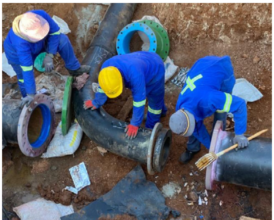
Working on the SE2 Phase 2 pipeline.
